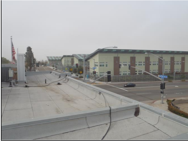
Southwest view from rooftop, institutional/school building
