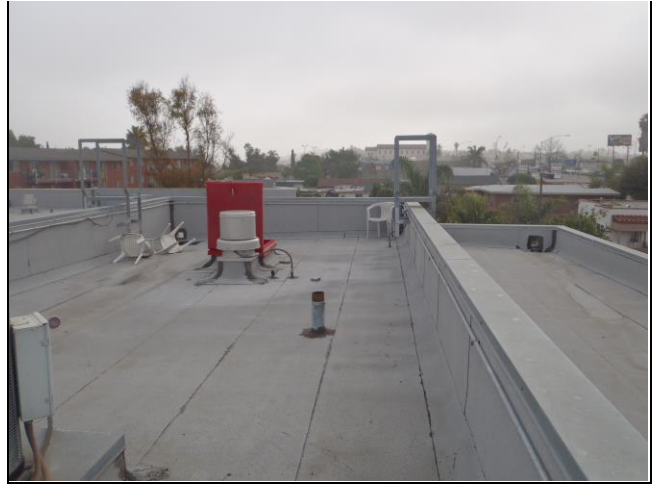
Northeast view from rooftop, surrounding residential area
