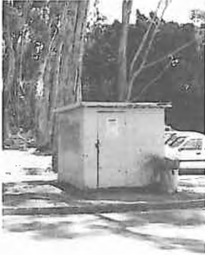
An existing grounds maintenance shed.
